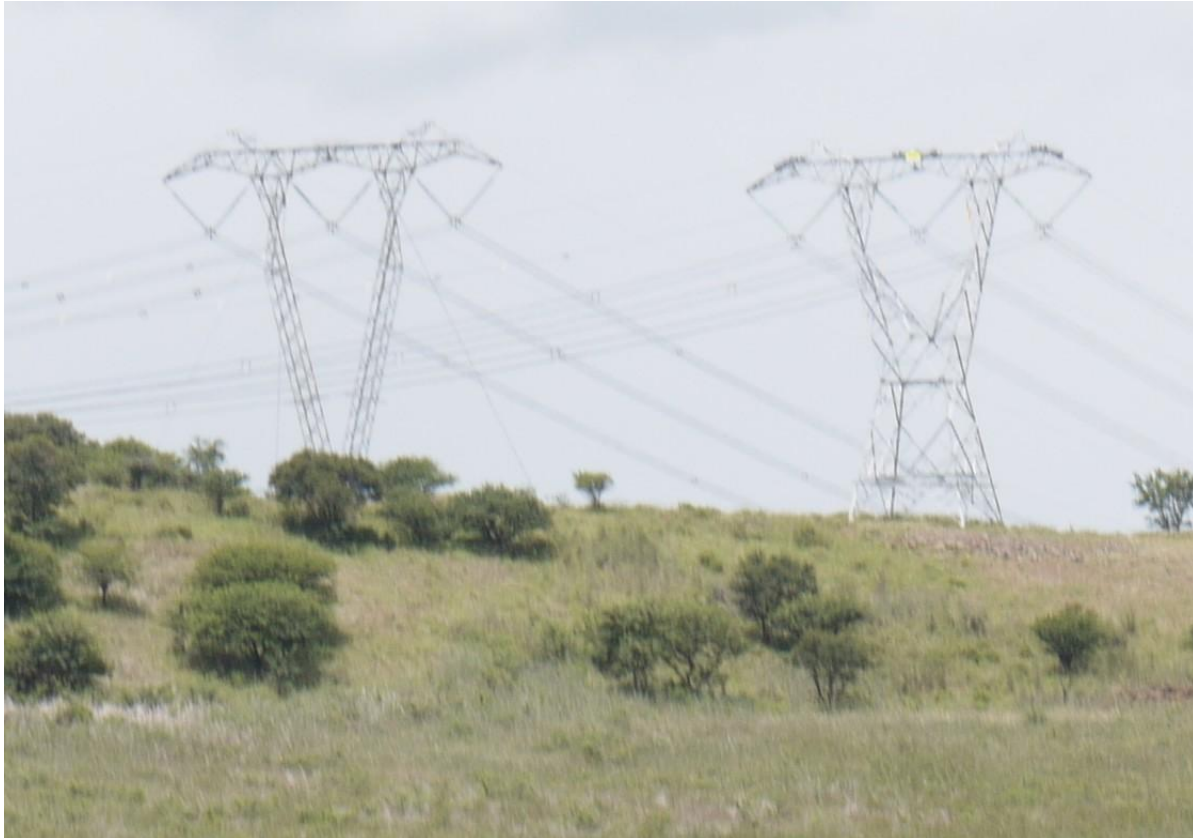
Plate 3, Guyed V tower on the left and Self Supporting Strain Tower on right are the two alternative 400kV alternative towers.
